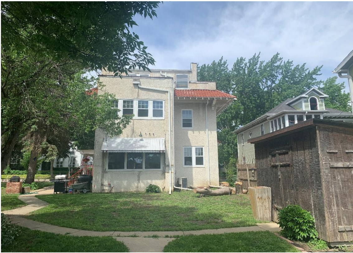
Above: Rear / East Façade
