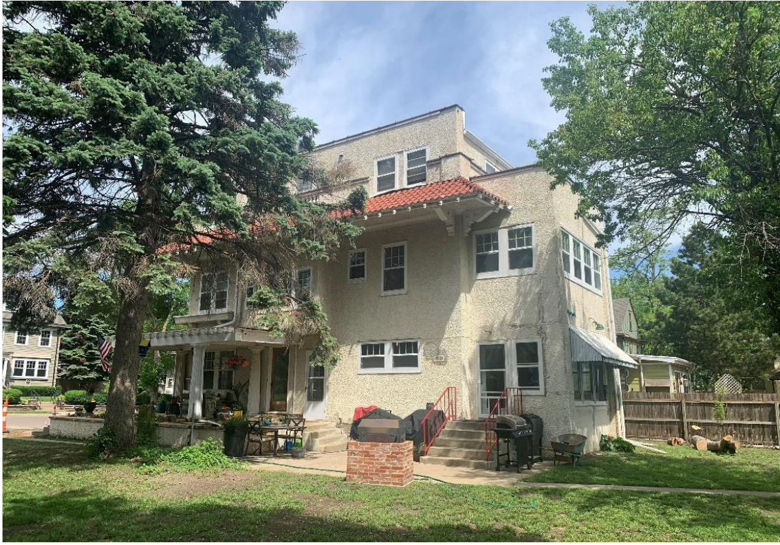
Below: Side / South Facade
