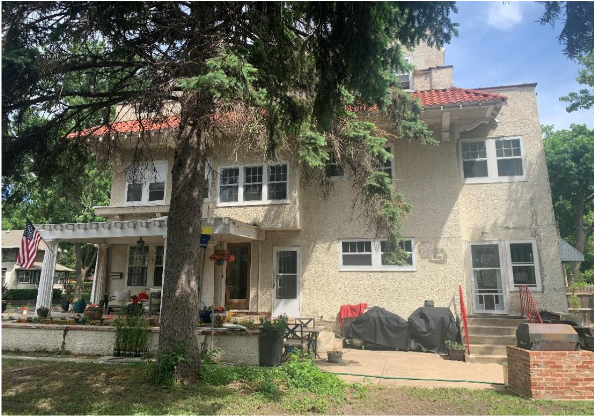
Above: Side / South Façade
