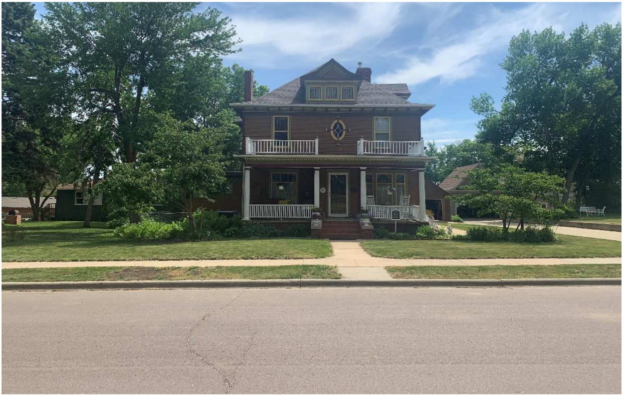
Above: Front / South Neighbor, West Facade
