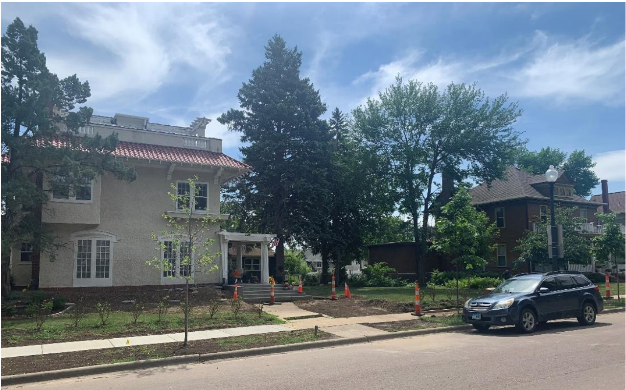
Below: Front / West Facade
