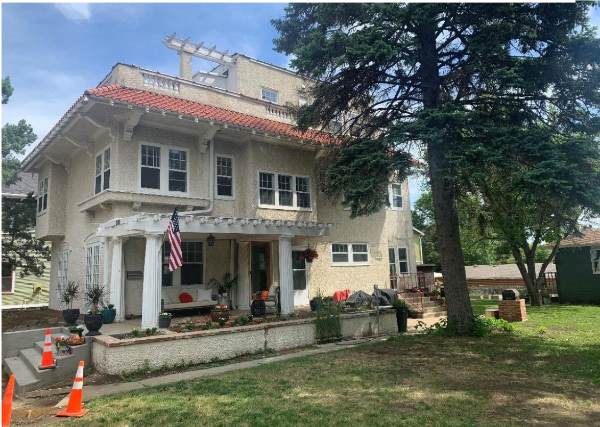
Below: Side / South Facade
