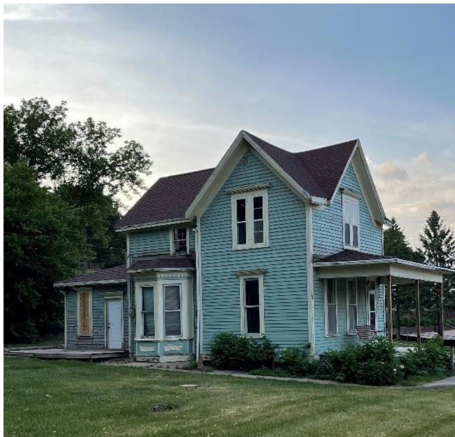
Below: 435 N. Spring Avenue – southeast view
