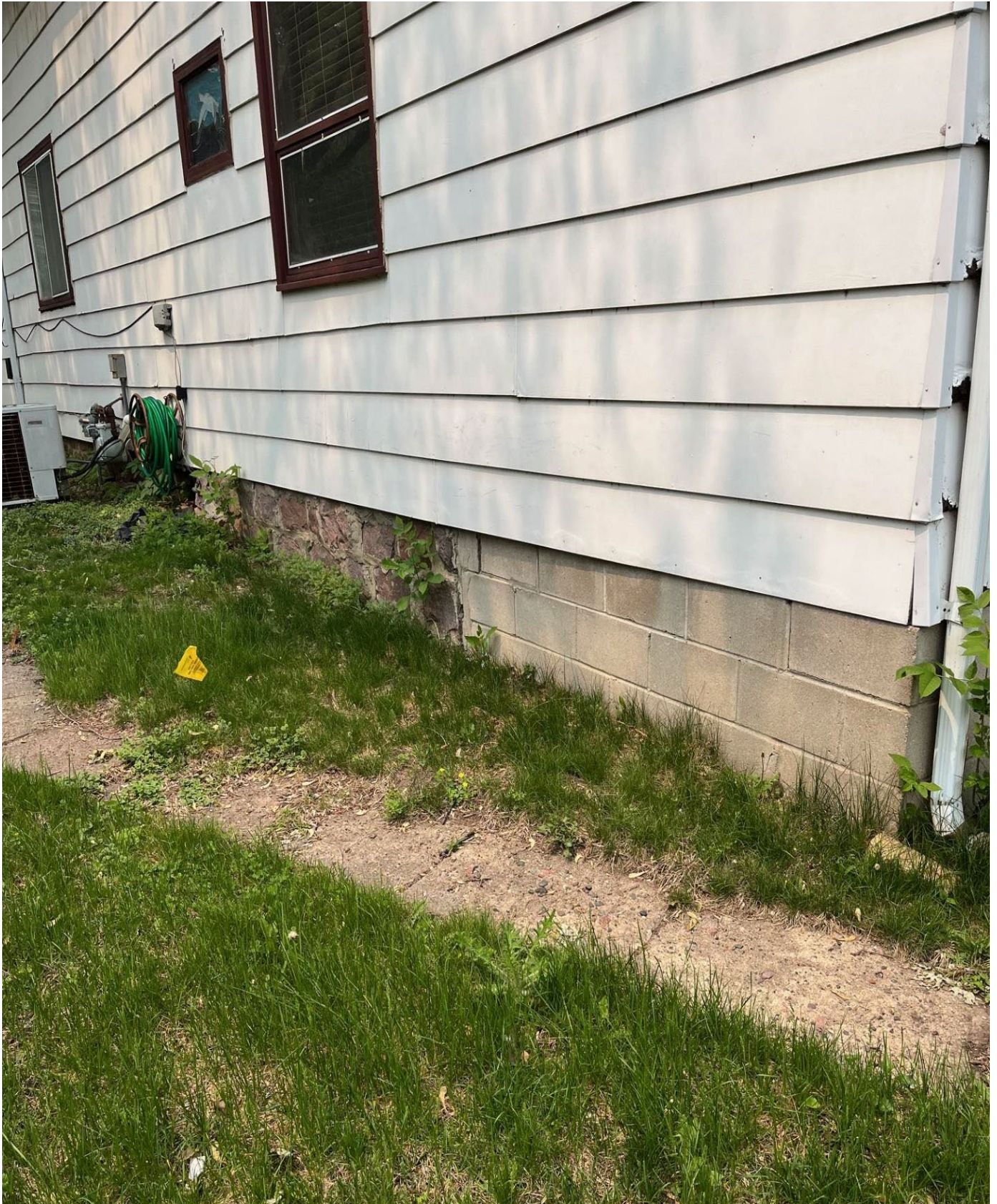
Below: 421 N. Spring Avenue – south facade
