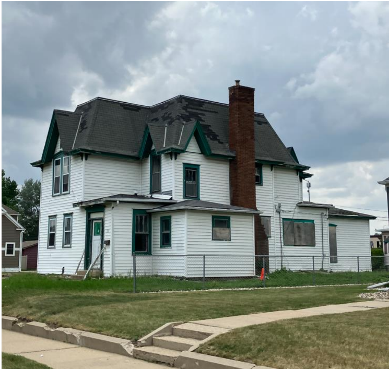
Above: 2023 Photo prior to vinyl siding and windows being removed.
