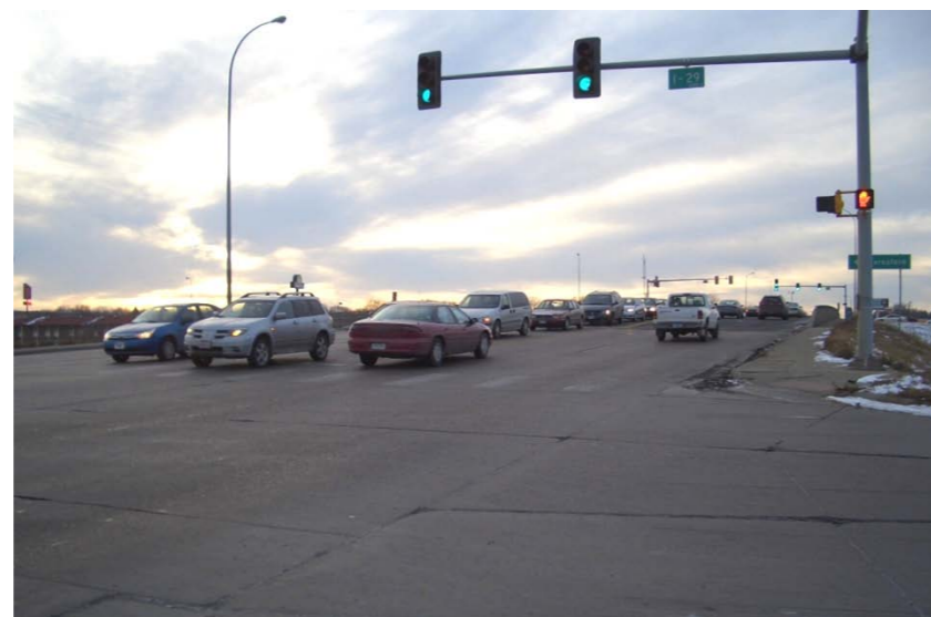
Photo shows sidewalk along 41 st Street at the I-29 bridge.
