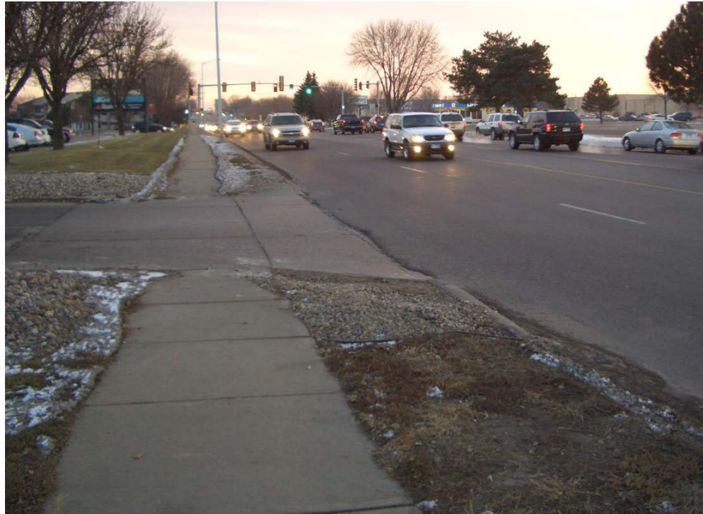
Photo shows sidewalk with boulevard along Louise Avenue.
