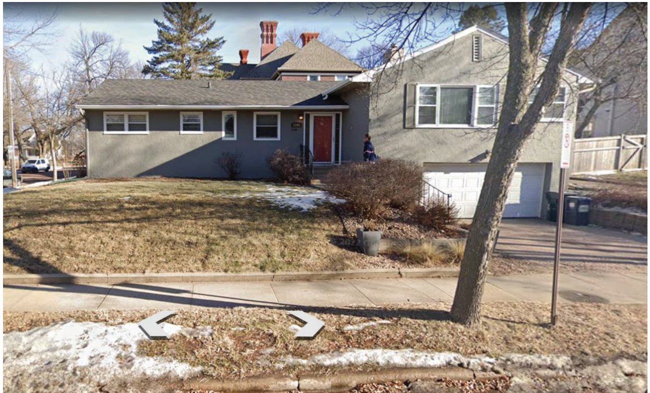
Below: 1200 S. Phillips Avenue. North of 1212 S. Phillips Avenue
