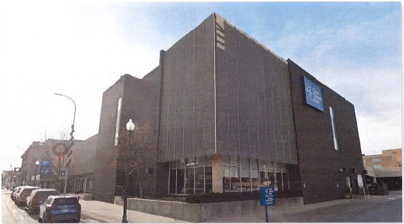
EXISTING BUILDING - Northeast view
