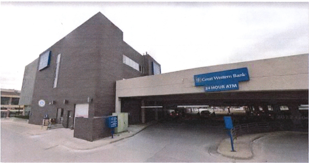
EXISTING BUILDING - Northwest view
