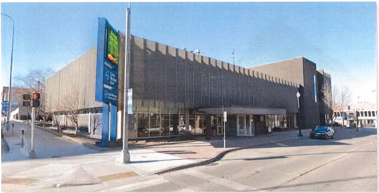
EXISTING BUILDING - Southeast view
