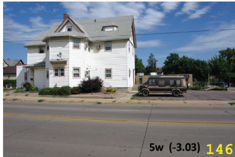
V/P: Land use conflict (residential/commercial/parking), No green, No buffer.
