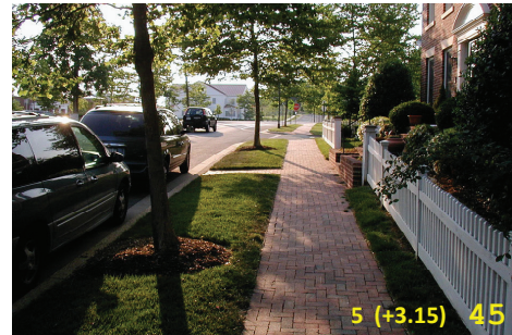
V/P: Pedestrian amenities (traditional r.o.w. section), Brick, Trees/green, Tight building setback, Picket fence defining private area, Separation/protection from moving traffic (shoulder area/parked cars), Well-maintained
