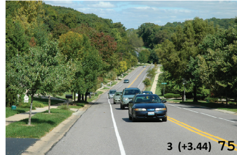
V/P: Road Diet (only 2 lanes), Bike/parking lane, Sidewalks, Separation of sidewalk from roadway, Trees in shoulder area, Green
