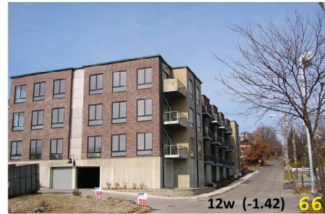
V/P: High-density residential, No green, No pedestrian amenities, No green, Cold concrete first floor
