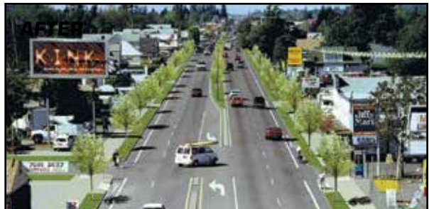
The complete streets concept: A combination of lane narrowing where possible, introduction of bike lanes, street landscaping, and sidewalk continuity can transform the appearance and actually improve the function of highly visible community streets. Often, the private sector responds to these public initiatives with better signage and upgraded development. (Photo from Michael Ronkin, Oregon Pedestrian and Bicycle Program Manager.)
