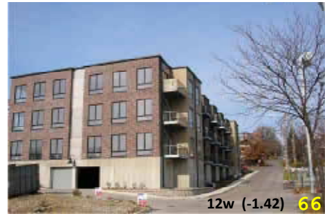
V/P: High-density residential, No green, No pedestrian amenities, No green, Cold concrete first floor
