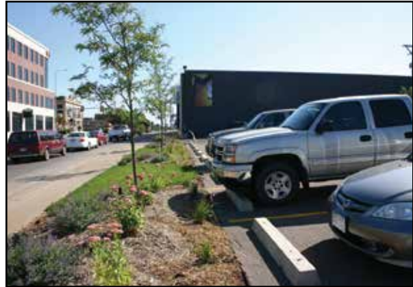
After street landscape buffer was installed.
