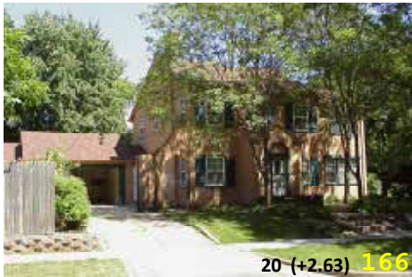
V/P: Traditional 1920's residential building, Green/trees, Tight front-yard setback, Recessed garage (not dominant), Well-maintained.
