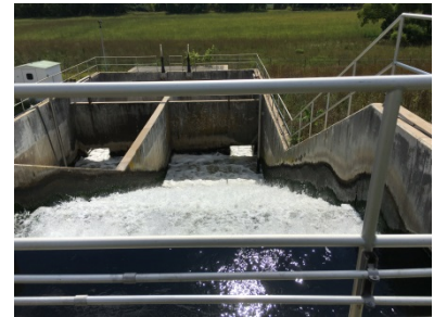
South Half of Cascade Aerator
