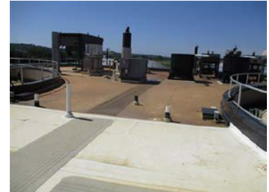
Energy Recovery Building Roof
