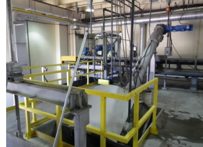
Rotary Drum Screen #1
