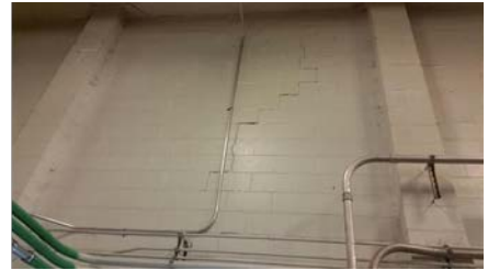
Interior Southwest Wall
