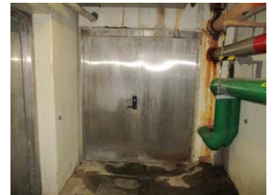
Interior South End of Tunnel
