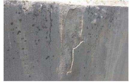
Parge/Skim Coating on the Clarifier Tanks
