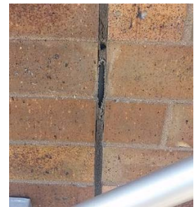
Sealant on Exterior Wall
