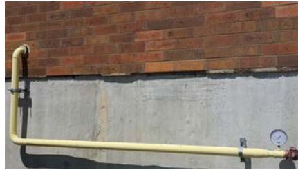
South Side Exterior Concrete Wall
