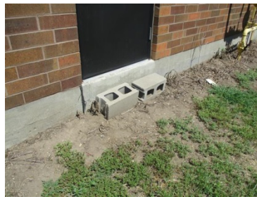
Rear Exit of Process Pumping Building
