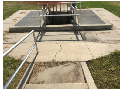
Sidewalks at Splitter Manhole #7
