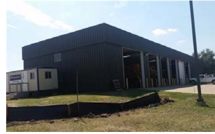
Exterior of Equipment Storage Building
