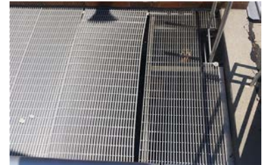
Grating on North Side of the RAS Building
