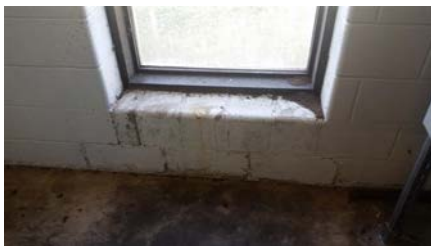
Window in Filter Building
