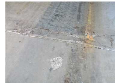
Concrete Floor at Overhead Door
