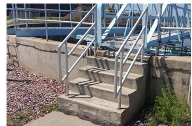
Concrete Steps and Sidewalk to the Final Clarifiers
