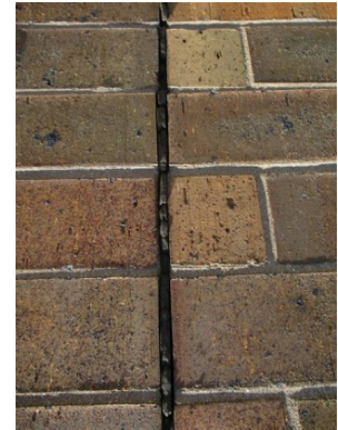
Masonry Control Joint Sealant
