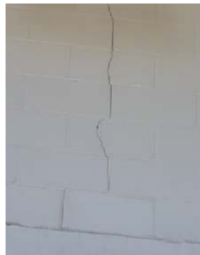
Interior Wall of the RAS Building
