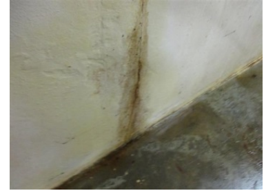
Walls in Lower Level Pump Room
