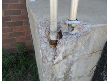
Stair Railings at NE Entrance
