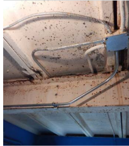
Adequate Ventilation – Supply and Exhaust Fans - Current NFPA Requires 6 ACH in Pump Rooms. If not they are then Classified as Class 1 Division 2
