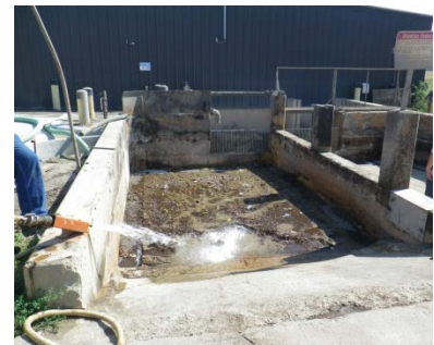
Septage/Vactor Truck Dumping Pit at EQ Basins
