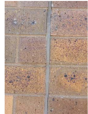
Exterior Wall Sealant of the RAS Building
