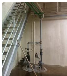
In-plant Pumping Building Interior Wall
