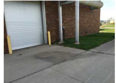
Overhead Door on Northwest Side of Control Building
