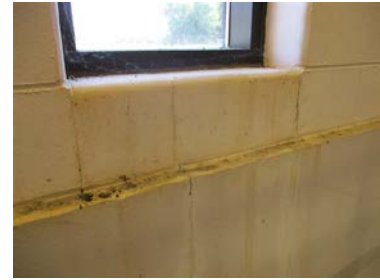
Masonry Control Joint Sealant
