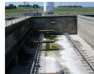
Aeration Basin #4A
