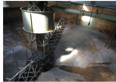
Gravity Thickener Mechanism
