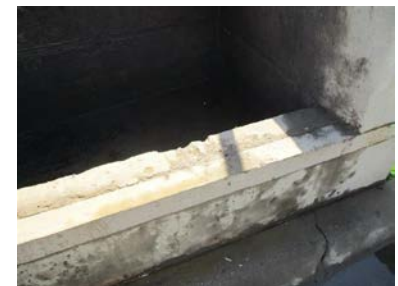
Concrete at Face of Dumping Area
