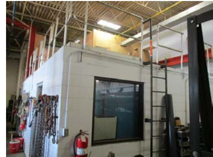
Mezzanine above Shop Office
