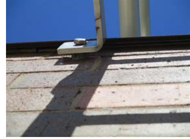
Roof Access Ladder
