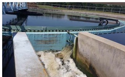
Paint and Coating of the Final Clarifiers
