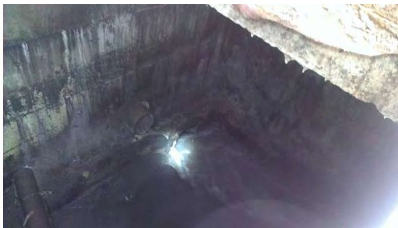
Figure 1: West Siphon Box
