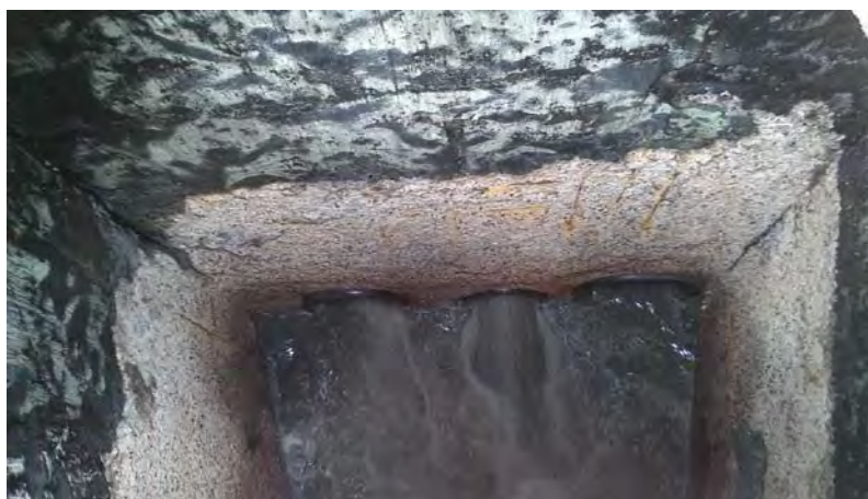
Figure 2: East Siphon Box
