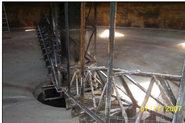
Figure 30 Gravity Thickener Truss Arms
