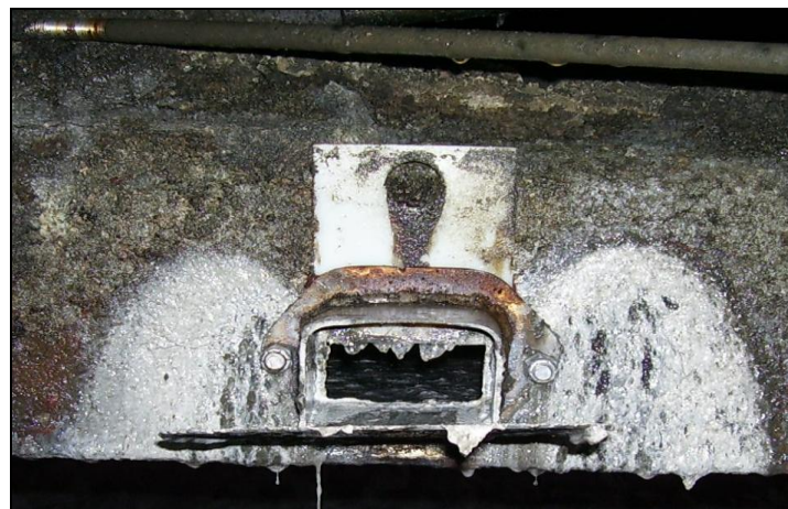
Figure 16 Trickling Filter Nozzle Detail
