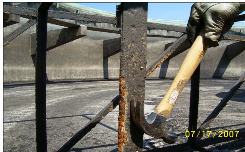
Figure 19 Final Clarifier #1 Truss Arms
