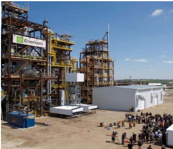
Photo #6: Enerkem Alberta Biofuels Facility, Edmonton, Alberta, Canada
