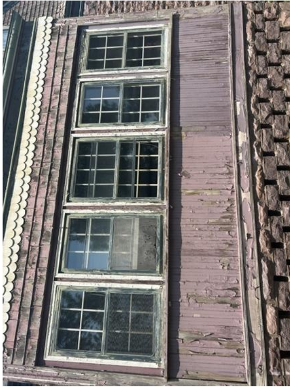
Window openings are inconsistent sizes, and paint/wood are failing throughout
