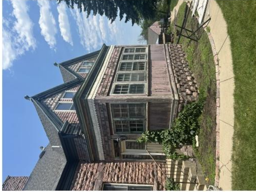
South elevation: sagging roofline, deteriorated shakes, and mismatched windows
