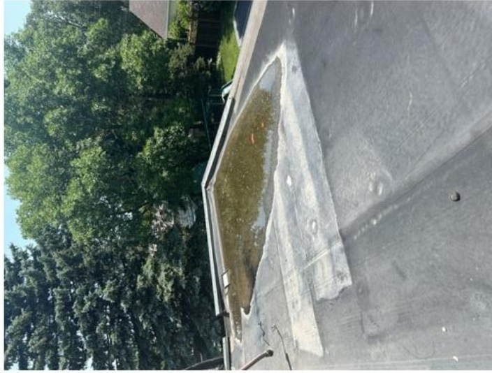
Flat roof is sagging and holds standing water, causing ongoing leaks
