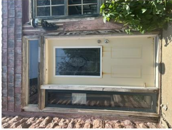
Exterior door and surrounding frame are rotted and failing
