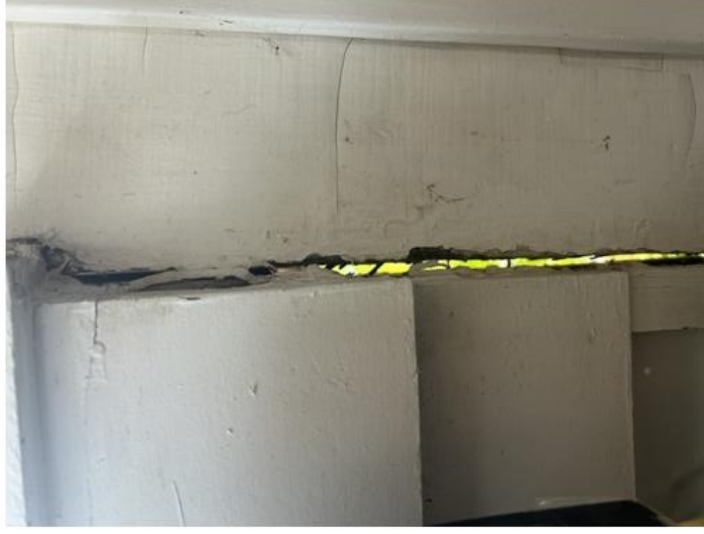
Daylight visible through the resulting structural gap
