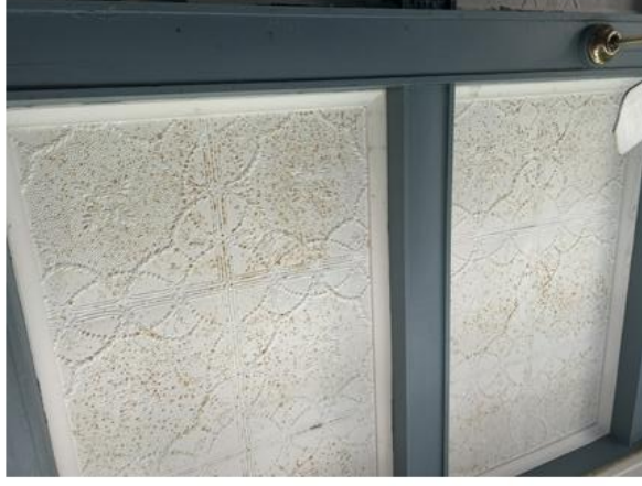
Interior ceiling shows water staining from the leaking roof above
