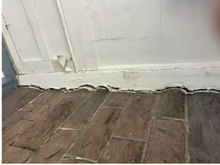
Structure has settled and is separating from the original house
