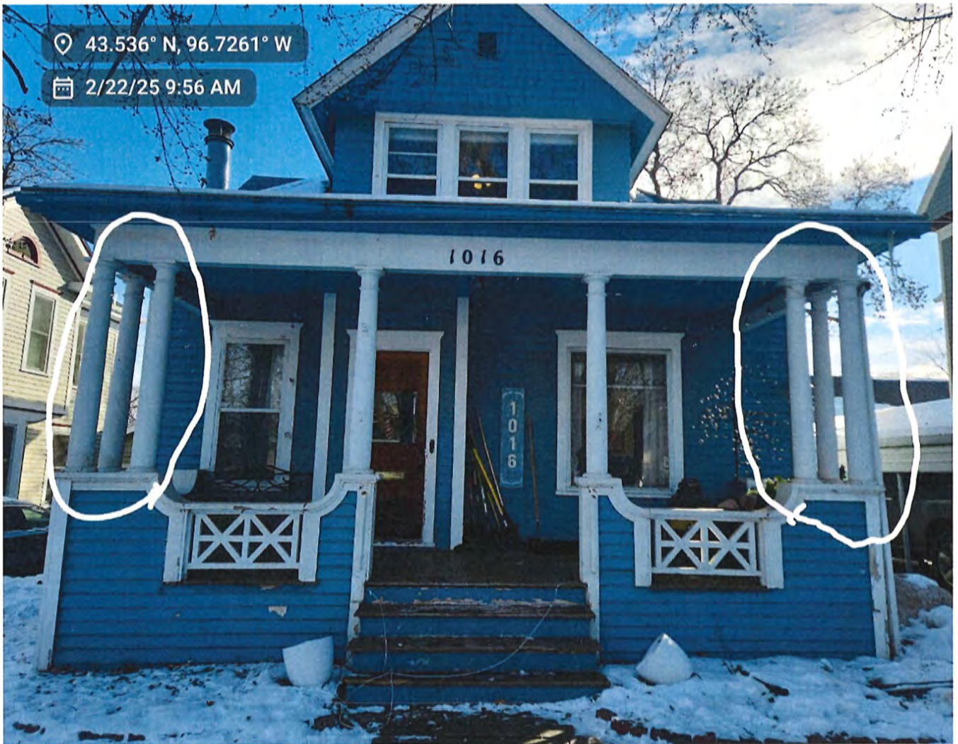
Above: West facade. Remove two of the three columns at each corner of the porch.
